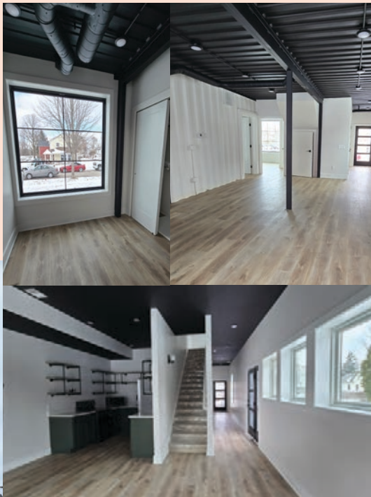
Top: Interior pictures of a container home show where containers were adjoined exposing the corrugated steel walls and ceilings, exposed duct work in the ceilings, and internal supports. Middle: The interior picture of the home constructed with prefabricated walls looks and feels like a typical stick-built home.
